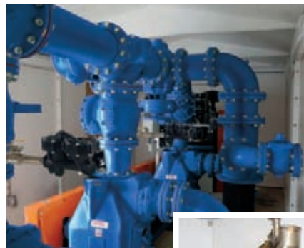
An Auto-Start package ensures pumping continues even when primary power has failed.
