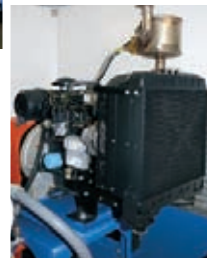
An Auto-Start package ensures pumping continues even when primary power has failed.
